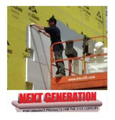
thickness of membrane and adhesive with standard hand trowel applications and allows simultaneous installation of drainage insulation. This feature makes waterproofing applications fast and easy, saving labor costs of 25% or more in efficient application of drainage insulation over vapor/air barrier membrane.
