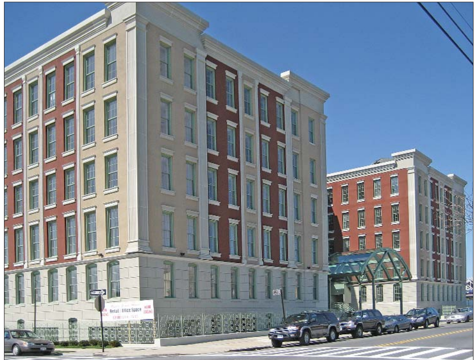
Steinway Piano Condominium Building, Astoria, New York
