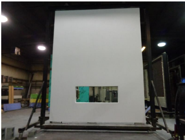
Photo No. 8 Completed installation of Exterior Cladding
