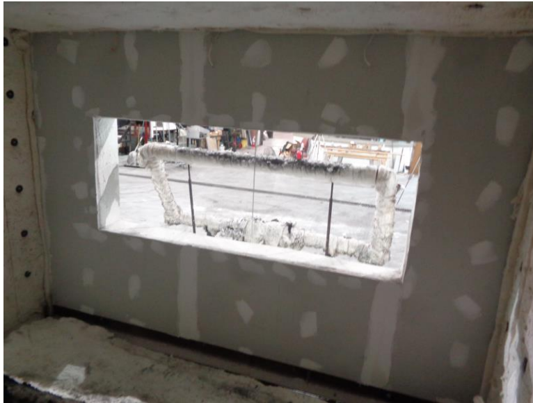
Photo No. 9 First Story Interior gypsum (Pre-Test)
