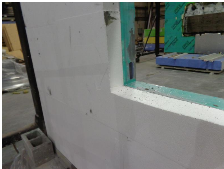
Photo No. 6 Completed Installation of Insulation
