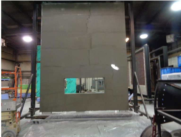
Photo No. 7 Installation of Exterior Cladding
