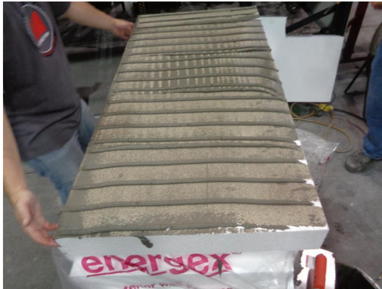
Photo No. 5 Installation of Insulation
