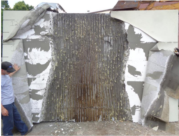
Photo No. 19 Exterior Cladding Removed (Post-Test)
