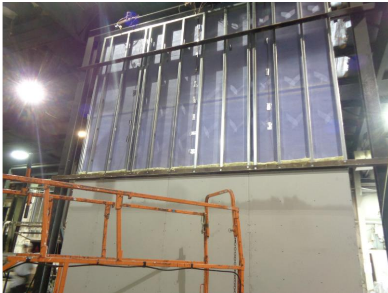
Photo No. 2 Safing Installation
