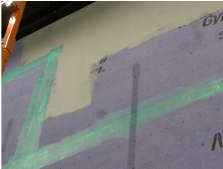
Photo No. 3 Application of AWB
