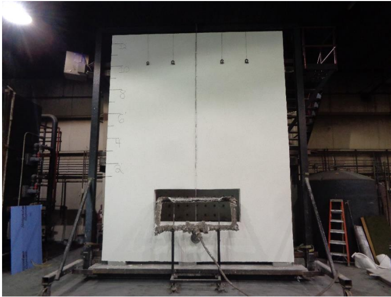
Photo No. 11 Finished Assembly (Pre-Test)
